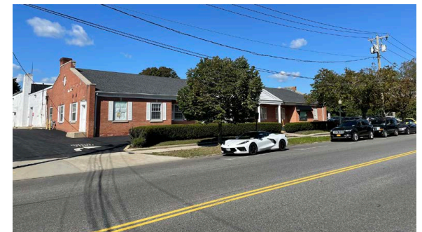
Vacant and underutilized buildings on Nugent Street
